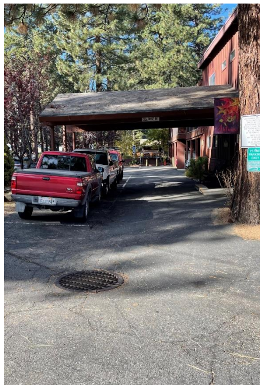
Photo 7 – Existing Porte Cochere
