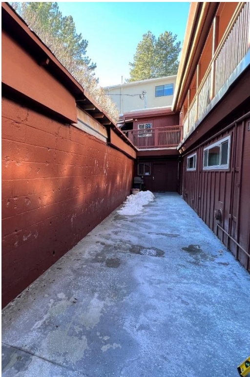
Photo 4 – Lower Retaining Wall
