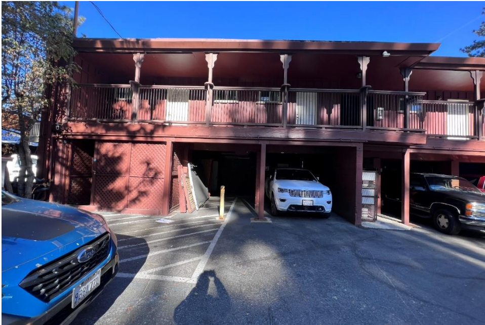
Photo 1 – Carport looking north
