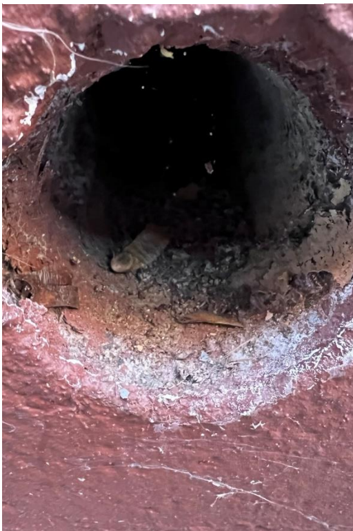
Photo 6 – Weep hole without evidence of moisture
